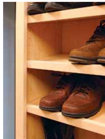
Simple shoe storage. A typical shelf design can be easily transformed into useful shoe storage by offsetting the shelf pins and turning the shelves upside down. The nosing extends to keep shoes from sliding off the tilted shelf.
