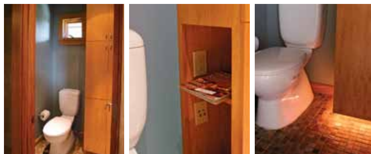
Accessorizing the water closet. A window high in the wall maintains privacy and provides natural light. Turned toward the toilet, the lower left side of the cabinet offers shelves for reading material, an outlet, and a data port. Rope light illuminates the toe kick as a night light.
